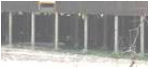
The pillars of Huma Betang was made from wood
