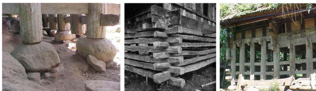
Figure 6 The base stone (left), the log-house construction (middle) and the pile-house construction (right).
